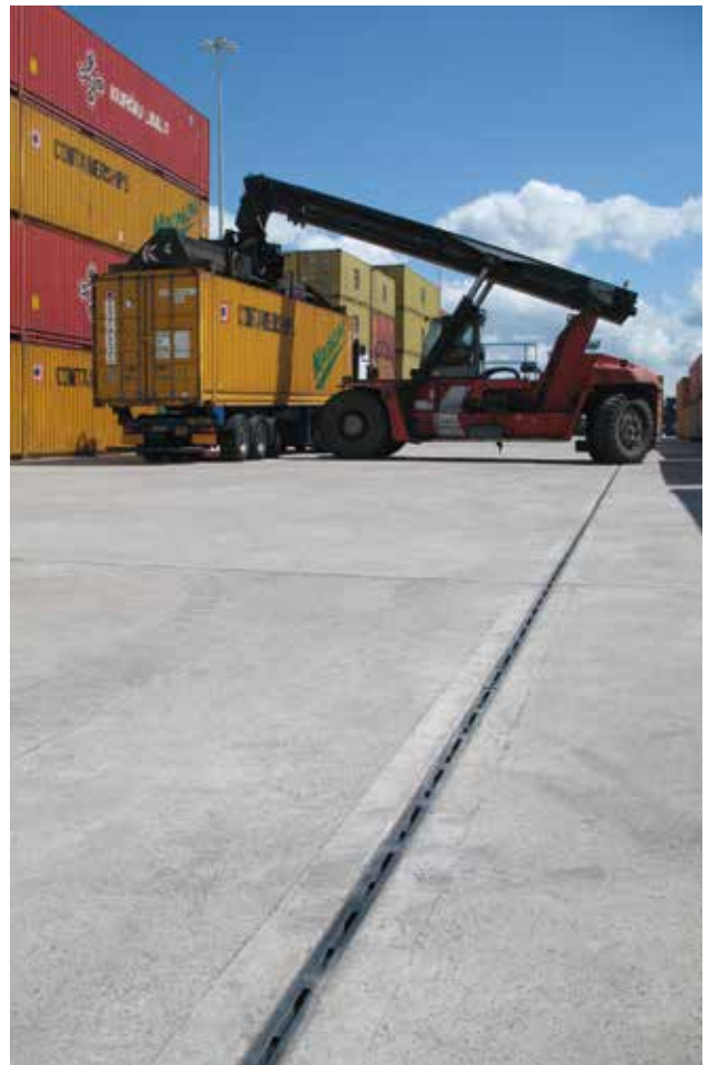
Teesport Container Terminal, UK
