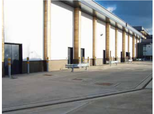
Installation in concrete surface
