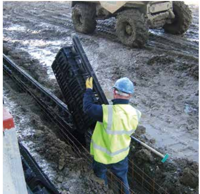
Lightweight elements, installed by one single worker.
