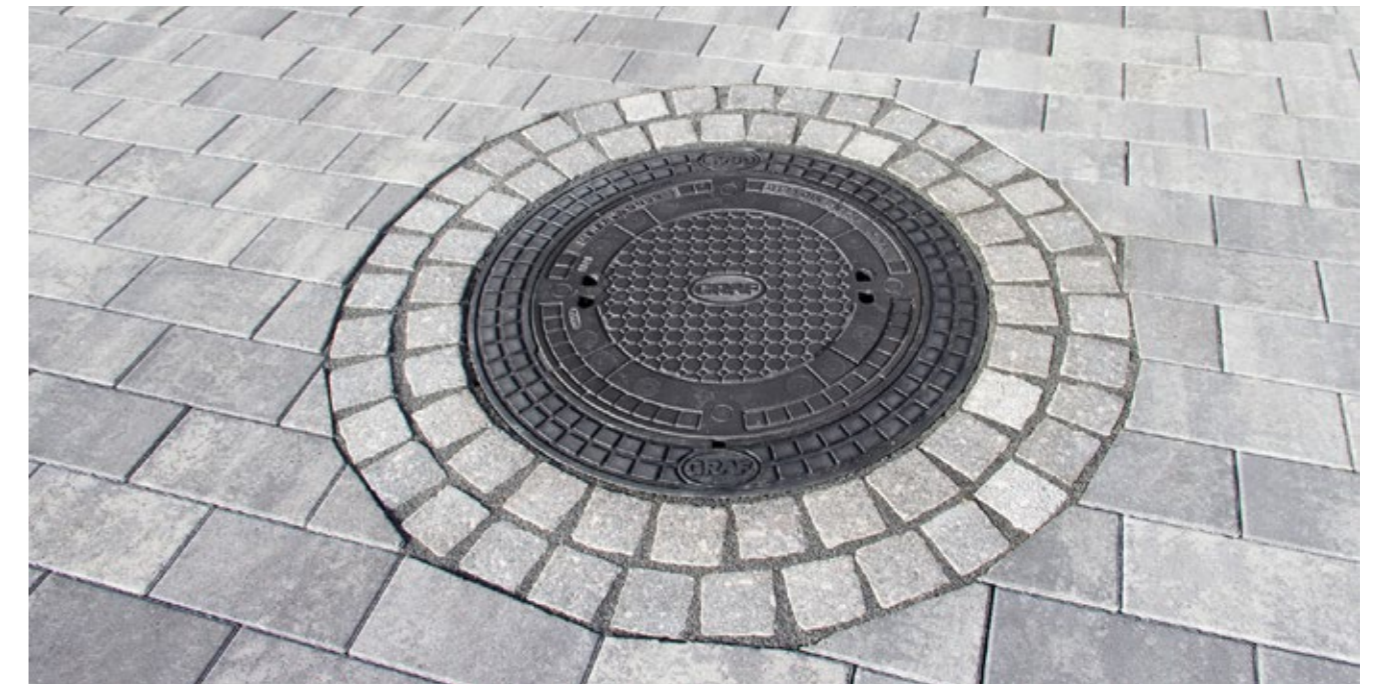
Solid lid suitable for vehicle/truck bearing – grated options available
